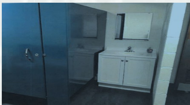
Women's bathroom after renovation
