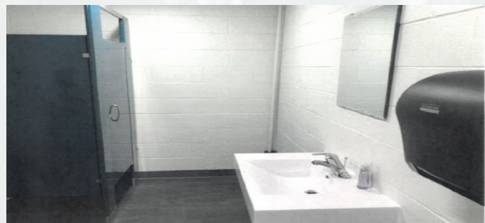
Men's bathroom after renovation
