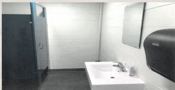
Men's bathroom after renovation
