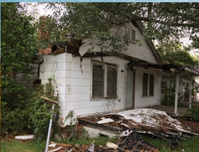
Home damaged by Hurricane Matthew to be torn down and rebuilt in Mullen, SC (across the street from job site pictured to the right).
