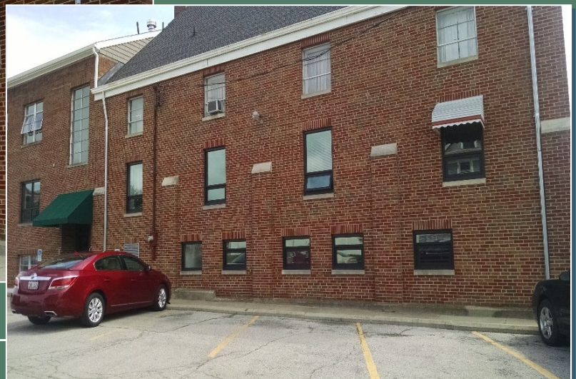
New Windows After Installation
