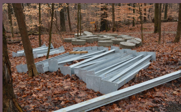
Bases and galvanized I-Beam posts to support the deck
