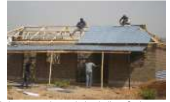
A three-room house being built at Gurku camp.
