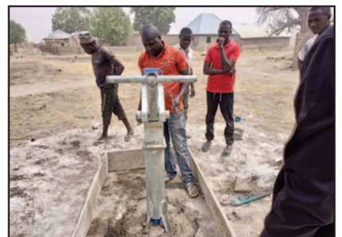
A handpump is installed on a borehole in Mussa Bri, Nigeria to provide fresh drinking water. Photo courtesy of EYN
