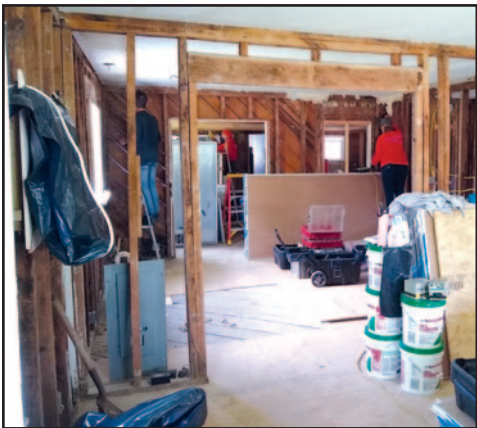
This Tennessee house, damaged in the August 2021 flood, is being gutted on the inside to prepare for rebuilding.
